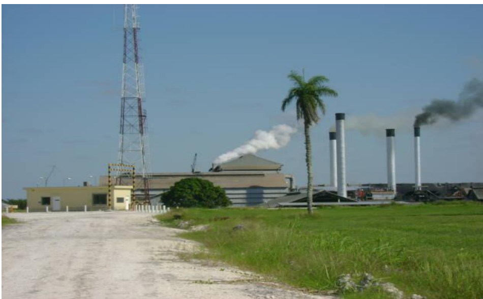
Figure 11 The Belize Sugar Industry factory (Orange Walk) in operation
