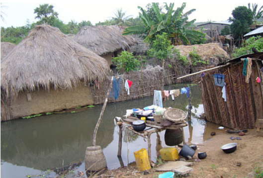
Flood damage across western Africa Photo: WHO
