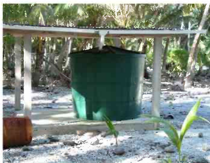
Water tank in Pukapuka
