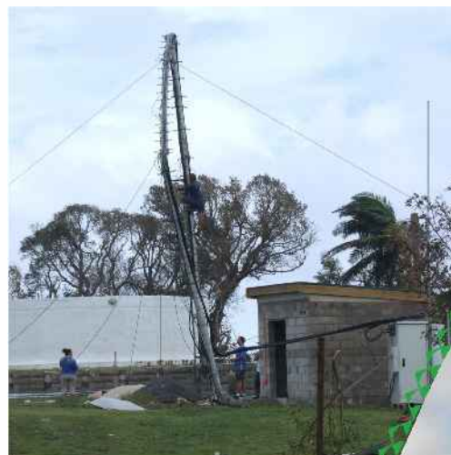
TCI Tower damaged in Aitutaki
