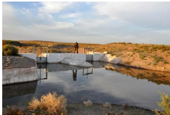
Repaired "Sharuashylyk" main canal. Photo: Katerina Yushenko/IINDP CBA
