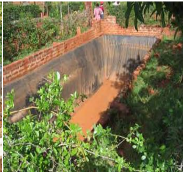
Reservoir built to capture run-off
